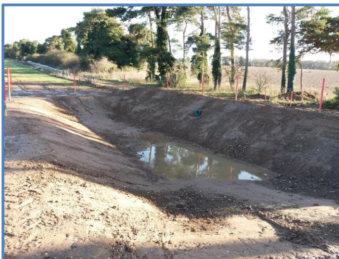
Figure 4. Silt trap (1) installed in December 2017.
